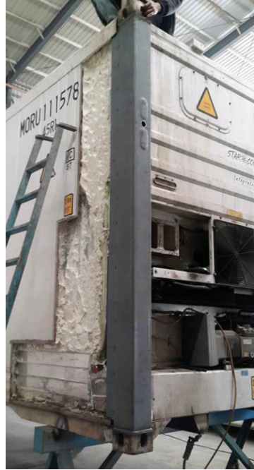
During repair. Very few machine parts need to be dismantled before the repair.
